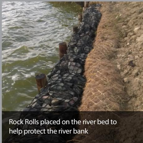
Rock Rolls placed on the river bed to help protect the river bank
